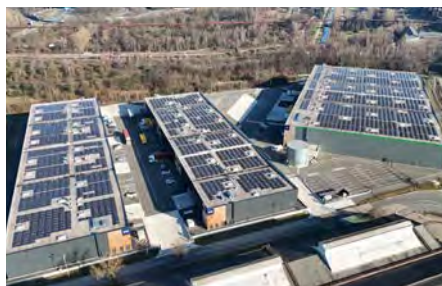
The park has three buildings with a total floor area of nearly 29,500 sq m (GARBE Industrial)
