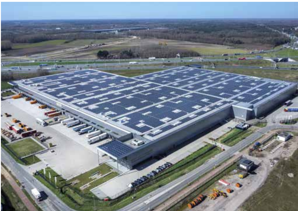
Rooftop power generation at Prologis Park Eindhoven DC3
